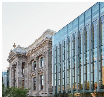
For enhanced building envelope performance, our curtain walls can be integrated with Vision Control®—Unicel Architectural's patented louvered insulating glass unit—providing dynamic control over daylight, solar heat gain, and occupant privacy.
