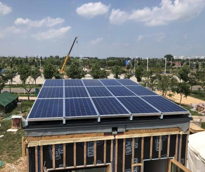
"A traditional photovoltaic panel converts about 20 percent of the sun's power to electricity – the rest being lost primarily through heat. With a BIPVT system, you can reclaim some of that heat with an air channel behind the PV to heat the house, thereby recuperating up to 70 percent of the sun's energy. Leveraging Unicel's advanced curtain wall and skylight technology, the TeamMTL house features a BIPVT front roof and a BIPV back roof that deliver high levels of thermal performance."
