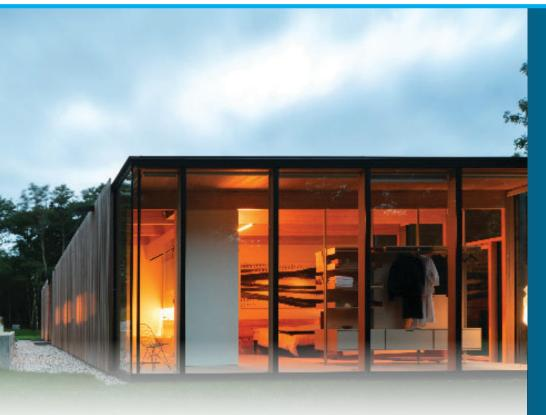
"The timber curtain wall solution with glazing and load-bearing columns was packed into readily transportable pieces and was assembled on-site within six days. A seamless, pragmatic and easy construction experience."
