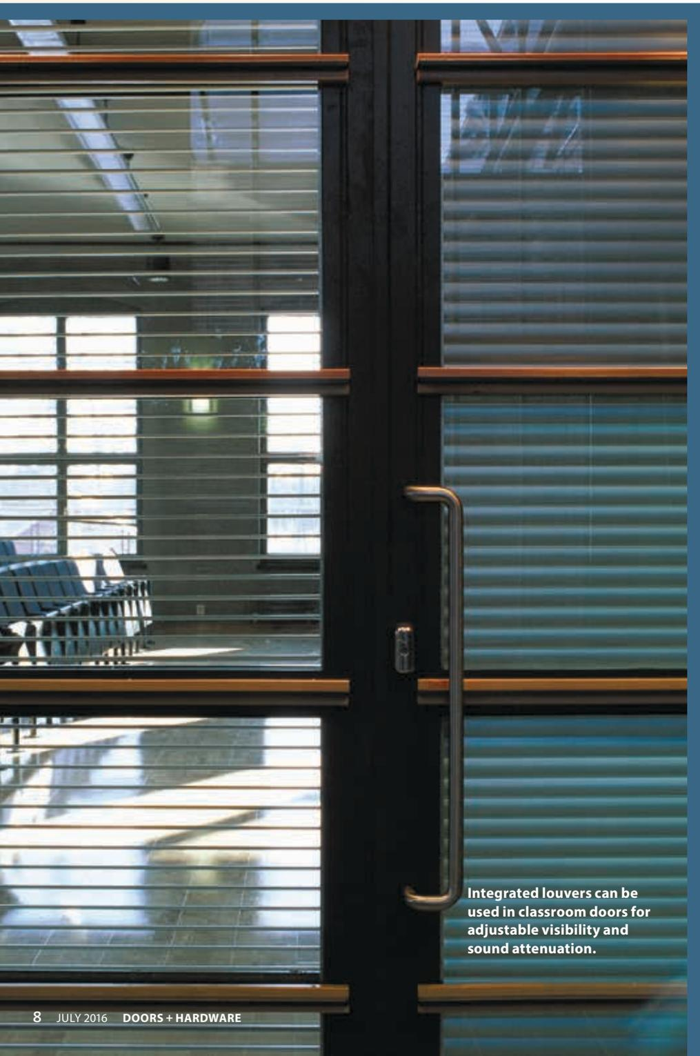
Integrated louvers can be used in classroom doors for adjustable visibility and sound attenuation.
