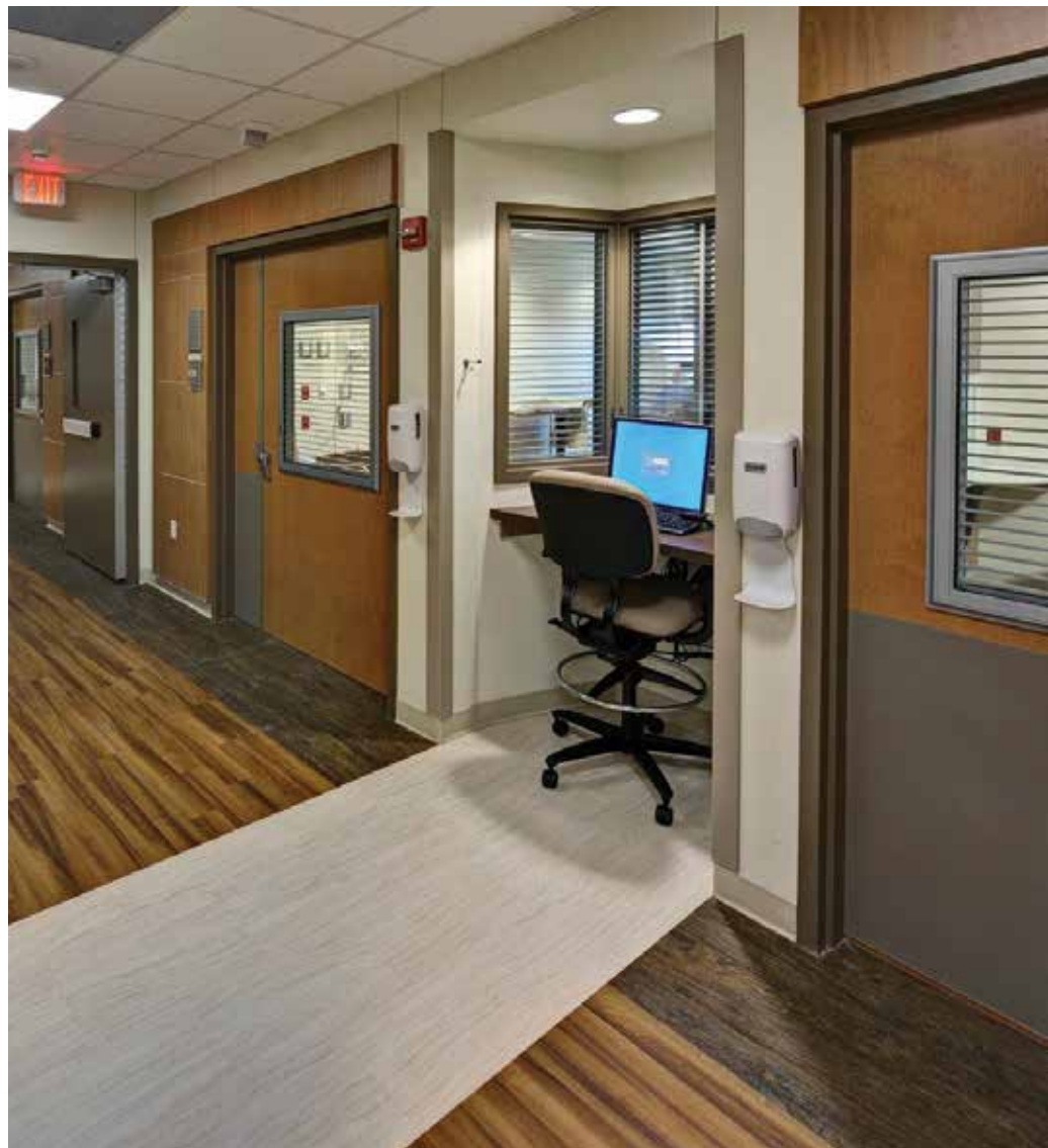
Sacred Heart Hospital, Pensacola, Fla. More than 70 integrated louver units were used in interiors doors and 160 in sliding doors to afford ensure a tranquil healing environment and acoustic privacy.
